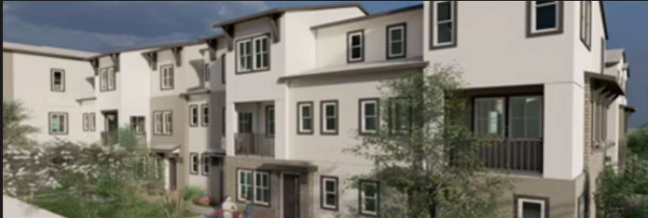
GROVE AVENUE - ONTARIO, CA
